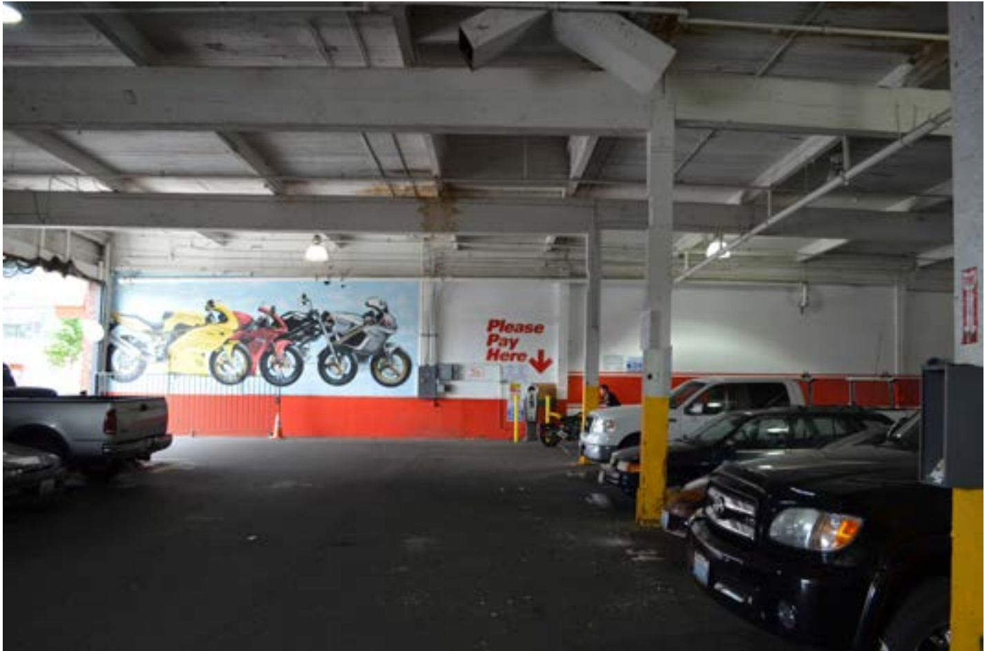
Garage Interior, July 2015
