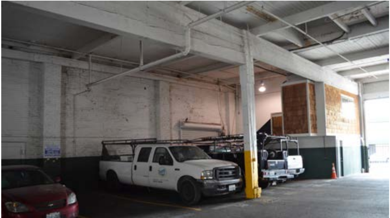
Garage Interior, July 2015
