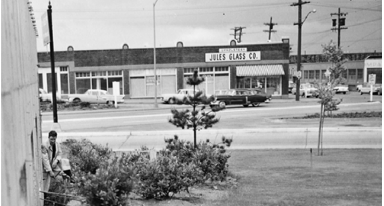
1962 photograph showing a partial south elevation. (Seattle Municipal Archives photo 71220)
