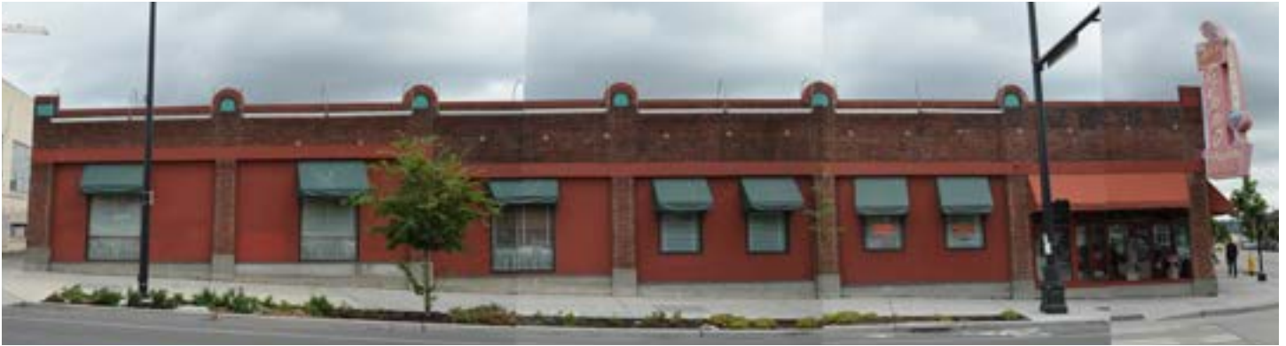
South Elevation, July 2015
