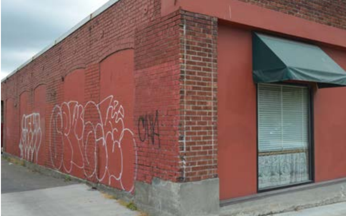
South-west corner at the alley, July 2015
