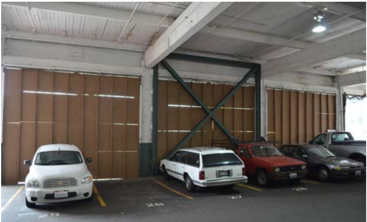
Garage Interior, July 2015
