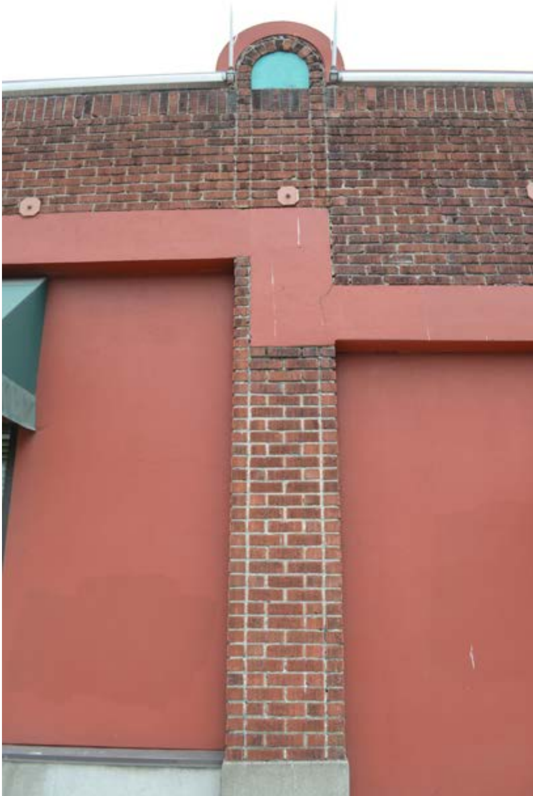
Facade Detail, July 2015
