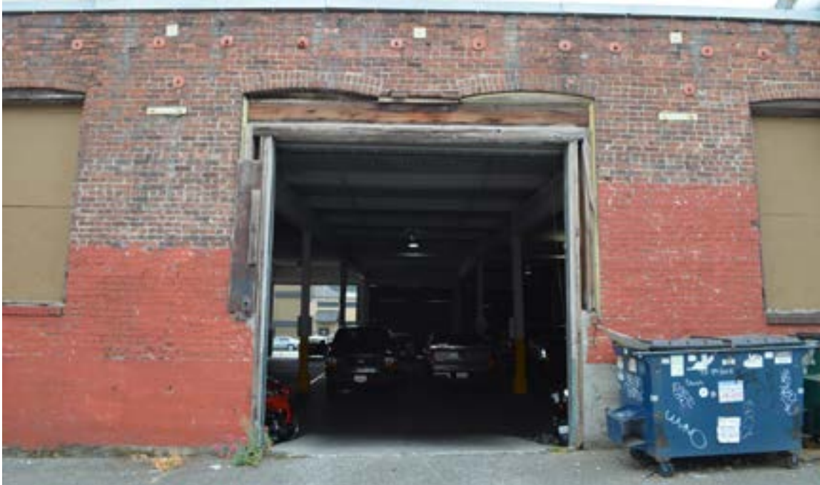
Alley facade detail, July 2015
