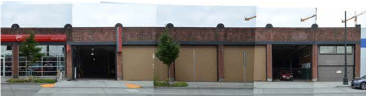
Partial North Elevation - Ducati window wall to alley, July 2015
