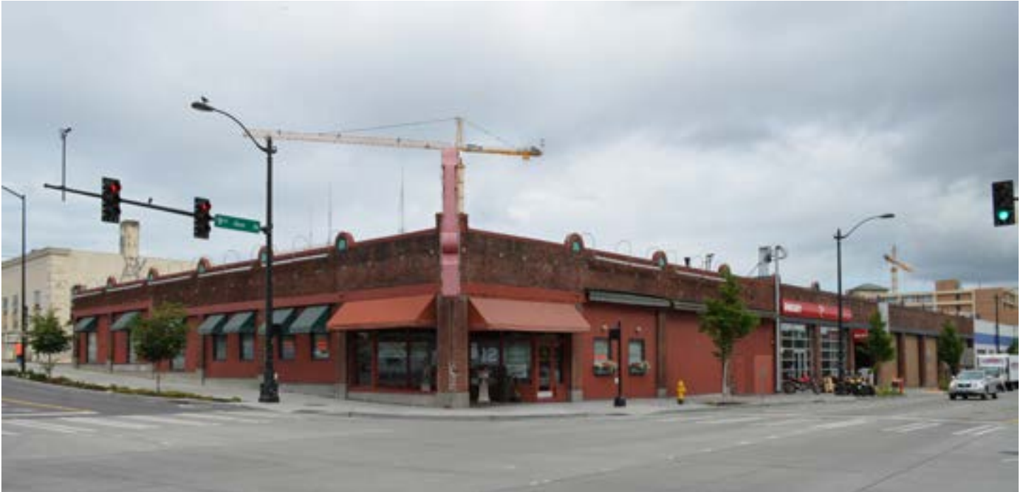
South-east building corner, July 2015
